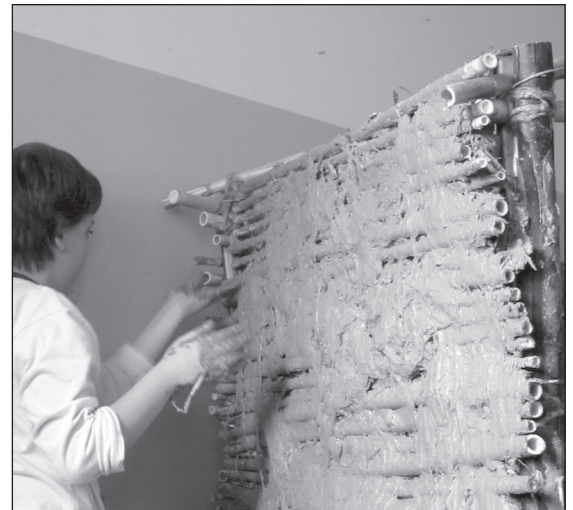
■ Fig. 8 Plaster preparation (clay and straw) on caning
