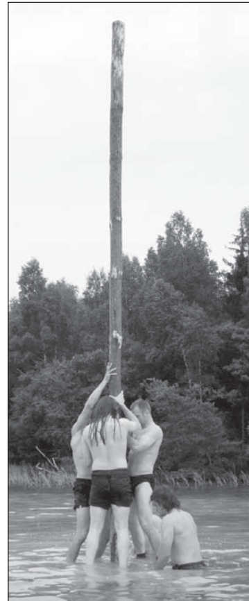
■ Fig. 15a The pile in a vertical position with three people standing on the movable wooden structure, ready to begin driving it into the lake marl (Photo: E. Pranckenaite)
