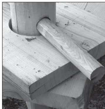
■ Fig. 7 Detail of the lower part of the movable structure
