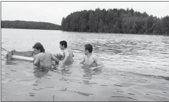
■ Fig. 12 Turning the wooden structure horizontally and sliding in the pile to be driven into the lake marl (Photo: E. Pranckenaite)
