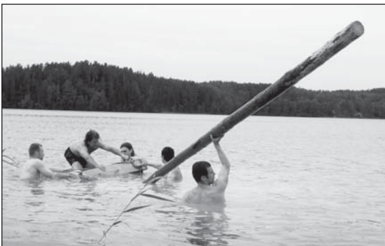
■ Fig. 13a Positioning the wooden structure and the pile in a vertical position (Photo: E. Pranckenaite)
