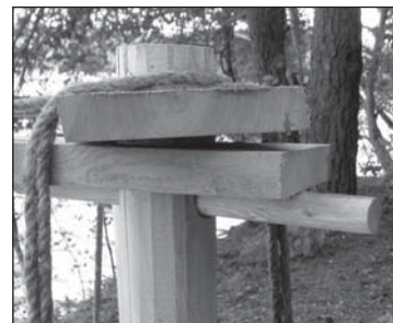
■ Fig. 6 Detail of the upper part of the movable structure
