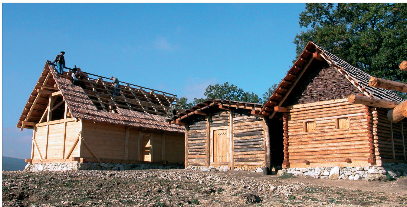
■ Fig. 11 The three most important wood house building techniques of the Iron Age: f.l.t.r. residential with threshold beams, wood-workers house in post technique and store house in log cabin technique.
