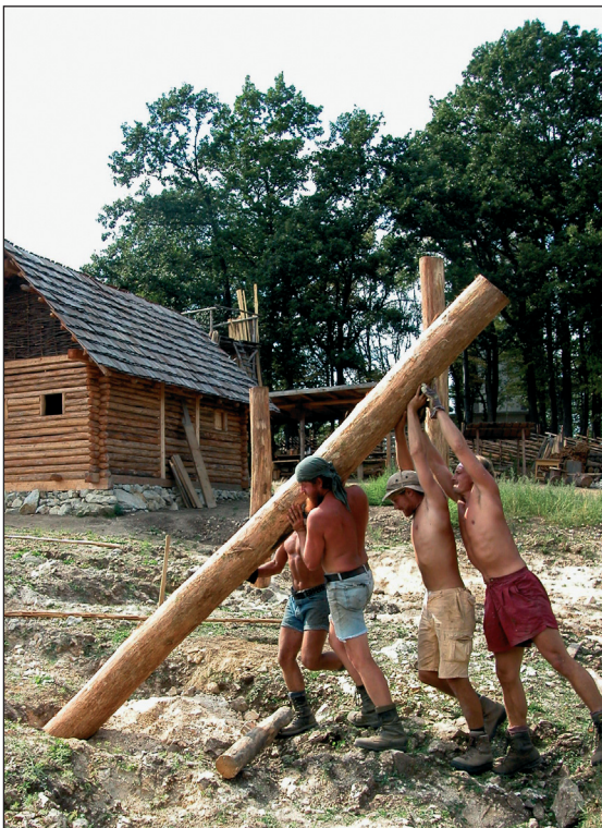
■ Fig. 10 The posts for the stable house were placed in pits in the ground. We erected them by hand.
