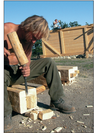
■ Fig. 8 Residential: the tenons and the according slots were worked out with chisels.
