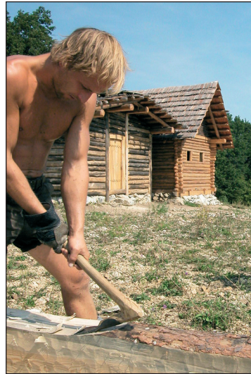
■ Fig. 7 The construction parts for the residential were shaped rectangular with iron adzes.
