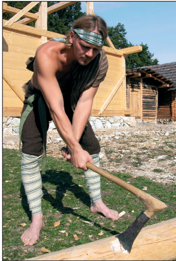
■ Fig. 5 The felling and the cutting of the logs was done with iron axes shafted on natural grown „knee-woods“ of ash and beech.
