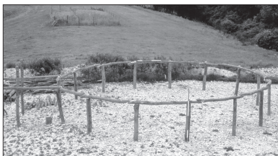
■ Fig. 3 The framework of the Balksbury house. Unlike the Maiden Castle house, its strength is drawn from the continuous wall plate attached to the uprights with simple mortice and tenon joints (in: Reynolds 1979, 94).
