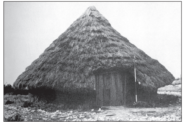
■ Fig. 1 Maiden Castle house: the completed structure. Set on the exposed spur of Little Butser this house has withstood hurricane force winds with impunity. Aerodynamically its shape is ideal. At no time is a flat surface presented against the elements (in: Reynolds 1979, 35).
