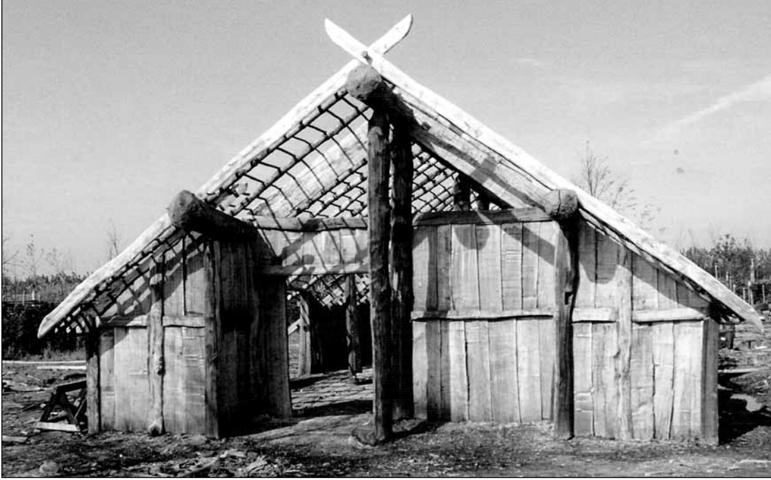
Fig. 2 The construction of the southeastern wall of Stein 29. Vertical placed planks between the outer posts. ■
