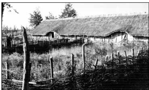
Fig. 6 The eastside of house Stein 29, one year before the fire. ■
