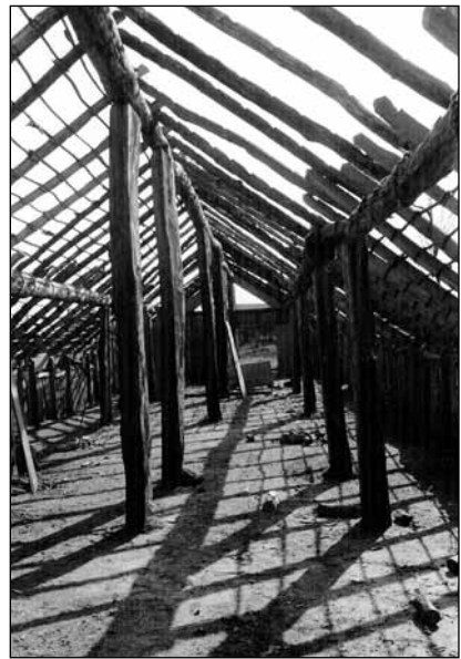
Fig. 3 The roofconstruction of Stein 29 with the short rafters from the ridge to the side plate and from the side plate to the wall posts. ■
